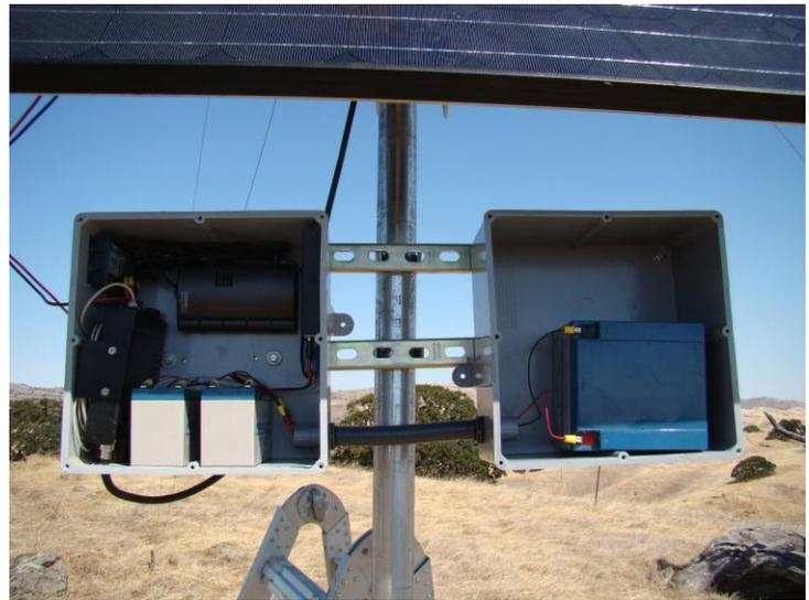
The above two pictures shows a solar install performed at Pacheco Pass. Instead of a standard console with display we used a weather Envoy in this setup. The pictures show two 7Ah batteries and one 26Ah battery with one 75 watt solar panel.
