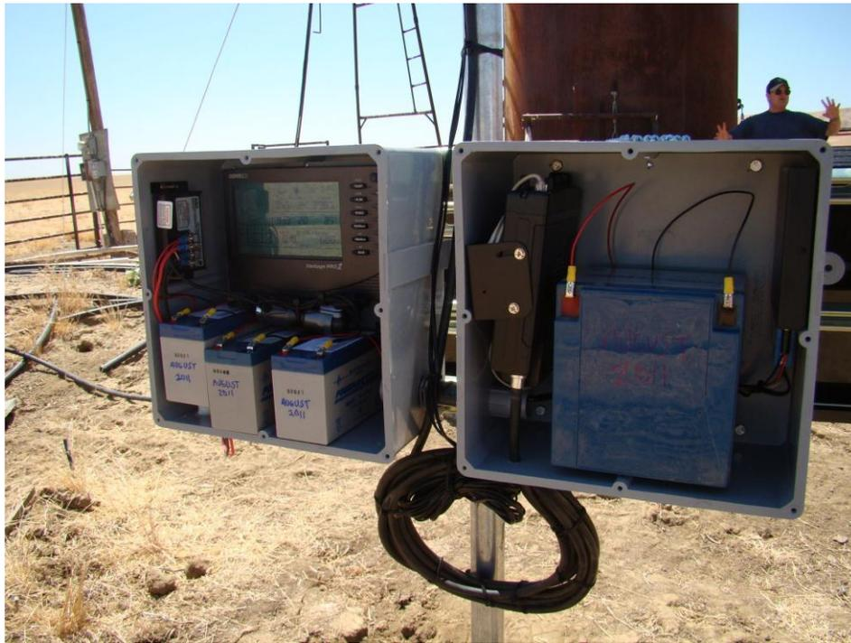
The above station is a solar station utilizing a full display console. It has 47Ah of batteries, 75W solar panel, and a 5A charge controller. Probably overkill but we were going for extreme reliability here. The bottom picture shows a similar setup with only 40Ah of battery capacity.
